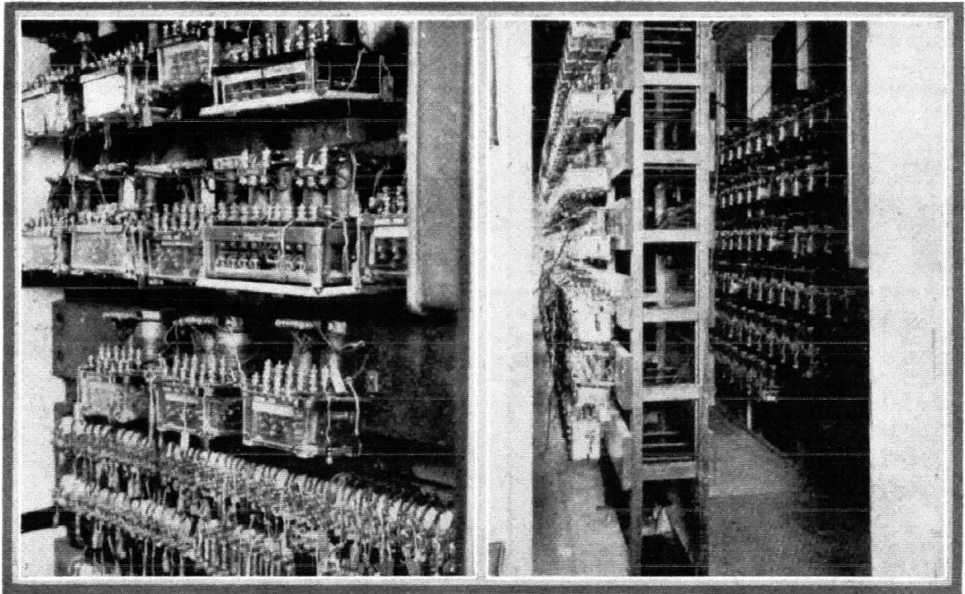
Interior of concrete relay house
